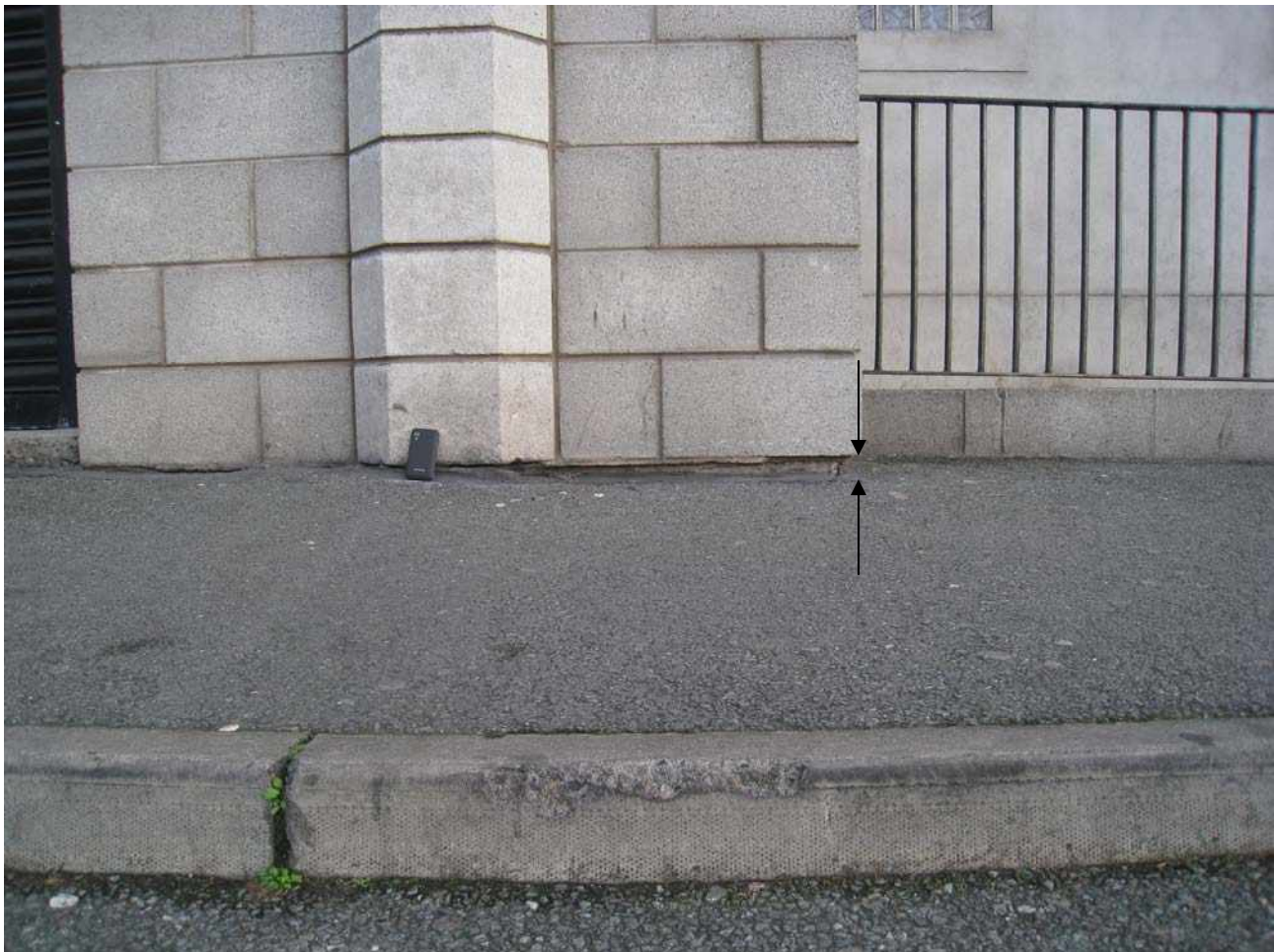
Fig PGGH_Dublin_006.10 differential movement of c. 5 cm
