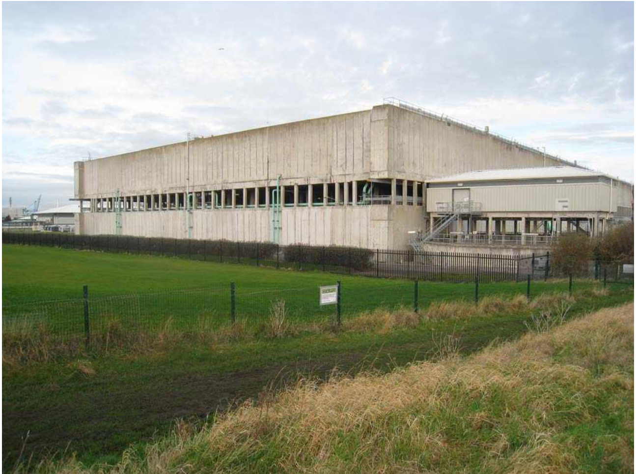
Fig PGGH_Dublin_009.2 Wastewater treatment plant
