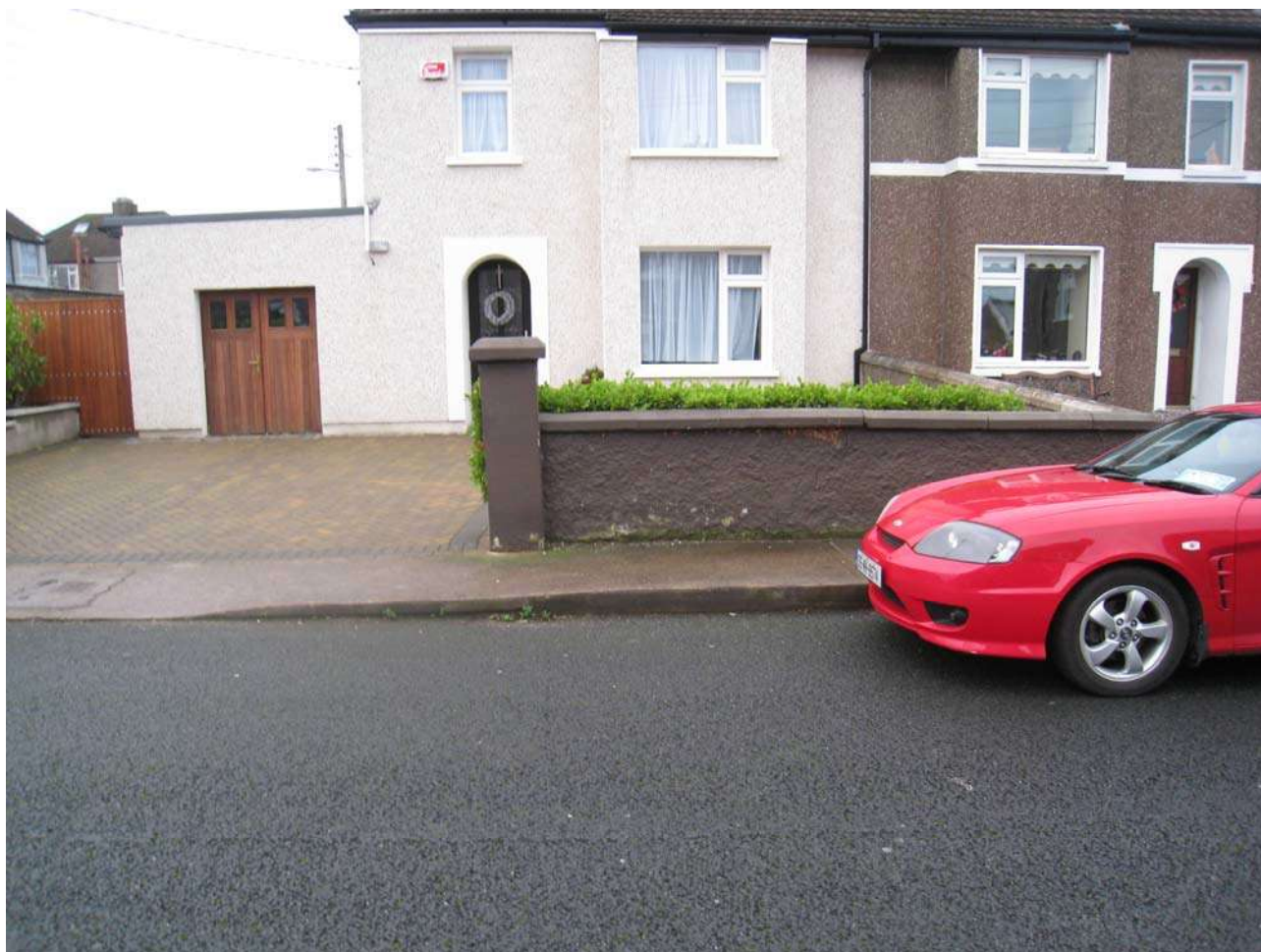
Fig PGGH_Cork_002.5 Typical newly underpinned and re-plastered house
