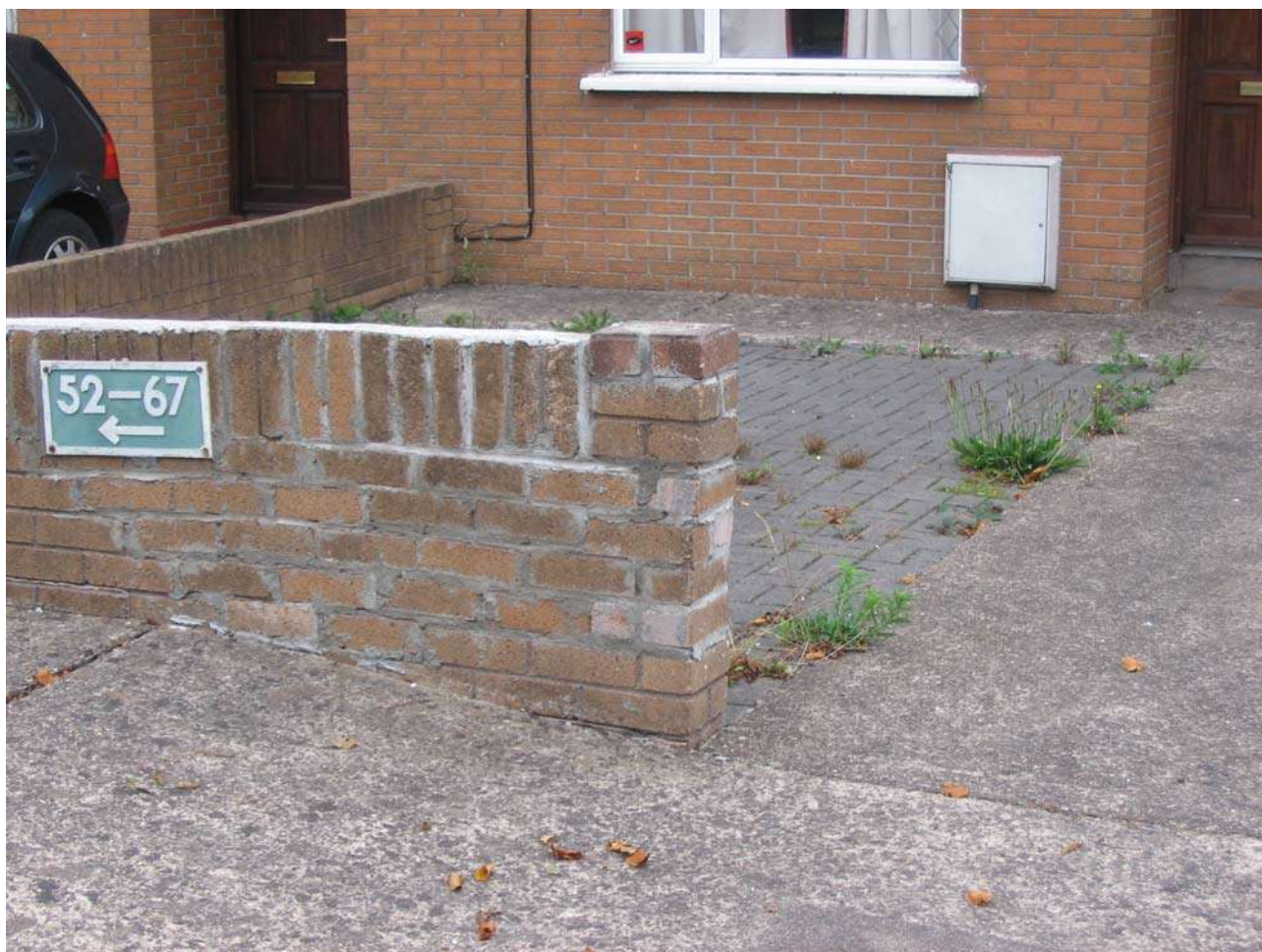
Fig PGGH_Cork_004.6 Repaired walls
