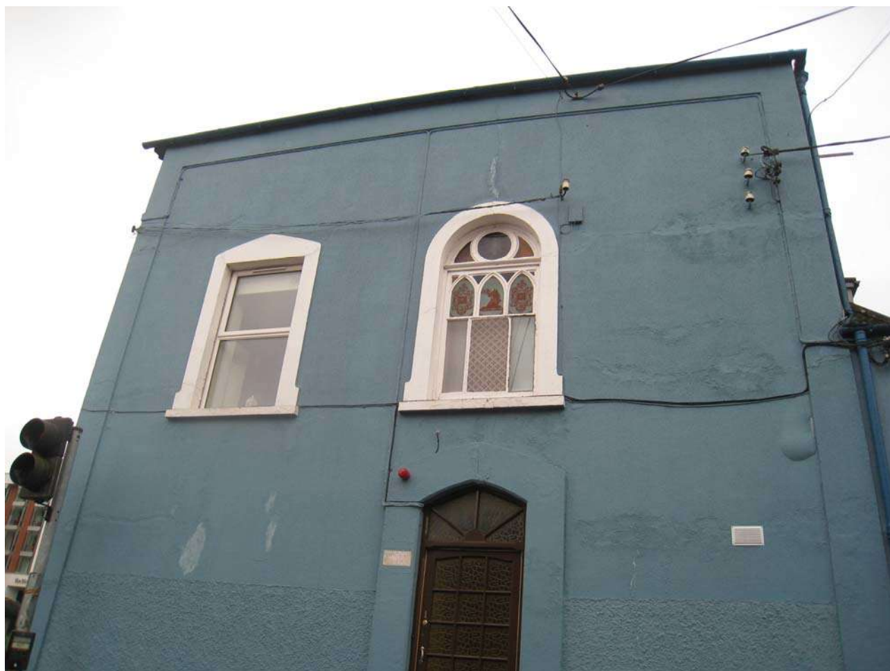
Fig PGGH_Cork_004.5 Repaired cracks in buildings
