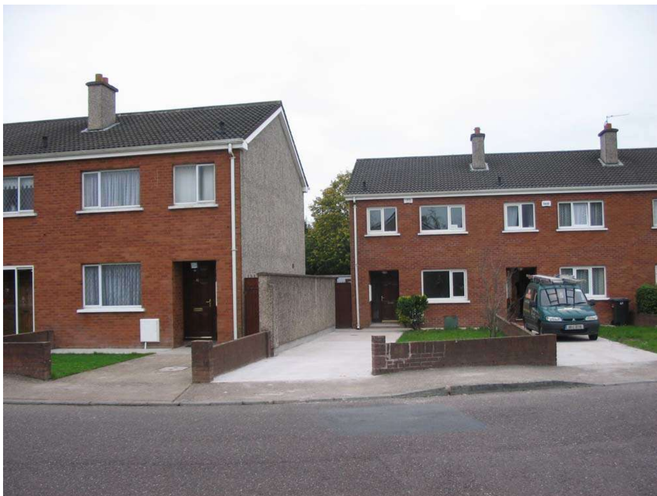
Fig PGGH_Cork_004.8 Recently underpinned buildings
