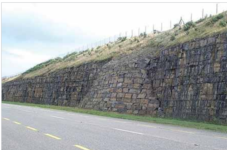
Figure 1-2: N17 Claremorris By-pass. A localised depression in the bedrock (infilled dissolution feature) was encountered in a steep sided rock cutting developed in horizontally bedded limestone along the N17 Claremorris Bypass. The soil encountered in the steepened side slope was retained behind a wall faced with limestone blocks in order to achieve a uniform geological profile within the rock cutting.
