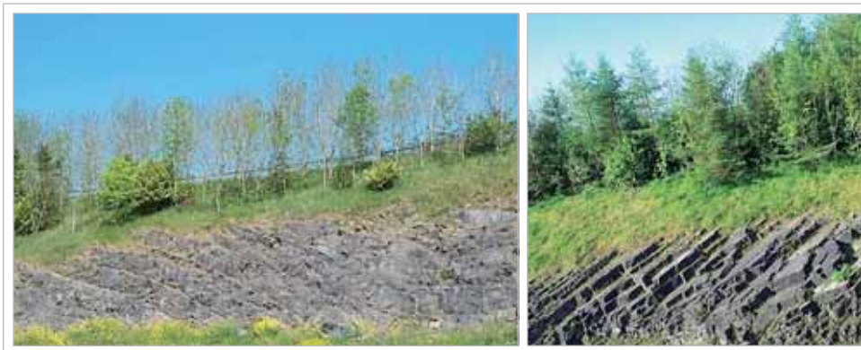
Figure 2-1: N4 Mullingar Bypass. The road cutting along the N4 Mullingar Bypass exposed a superb anticline fold in the Carboniferous limestones. As traffic enters the cutting, limestone beds dip one way and then level out at the top of the cut before dipping away in the opposite direction. This excellent visible demonstration of simple geological phenomena such as beds and folds was for a period rendered invisible by roadside planting.
