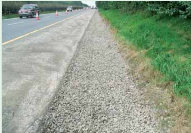
Figure 5-9: Example of a French Drain on M4
