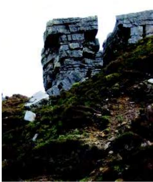
Plate 4.4 Potential toppling failure at Monesk on the Cavan/Leitrim border, also known as Englishman's Mountain. (Photo – Xavier Pellicer, GSI)
