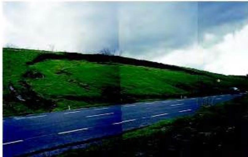
Plate 4.2 Slope failure in a glaciolacustrine deposit.
