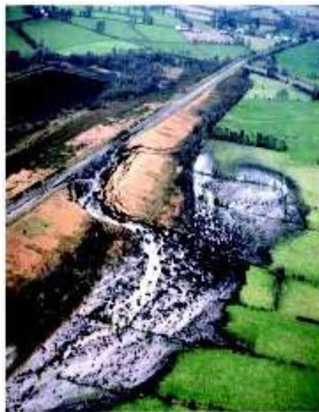
Plate 4.3 Slide on the Grand Canal, near Edenderry (Pigott et al., 1992)
