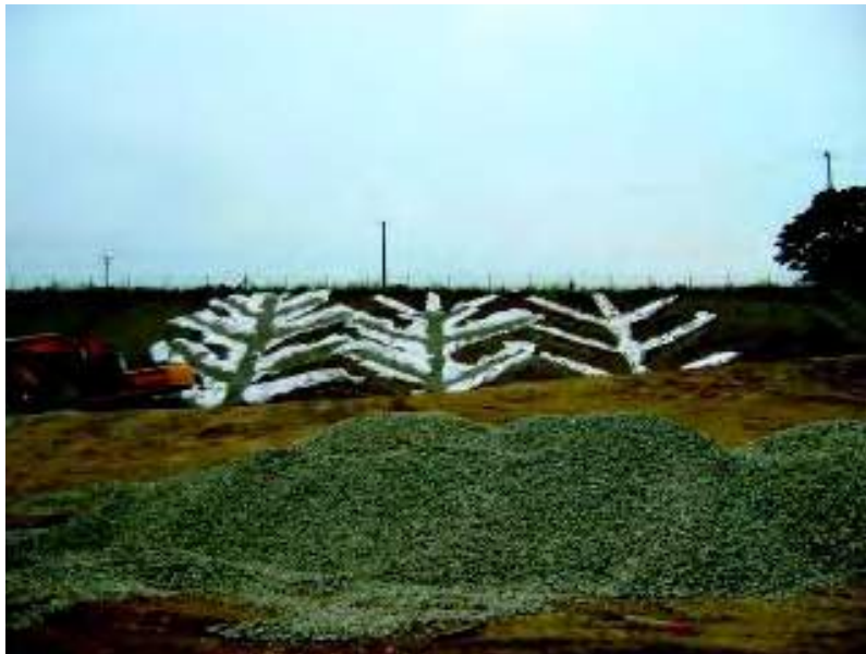
Plate 4.1 Herringbone drainage system being installed in cut slope of glacial till.
