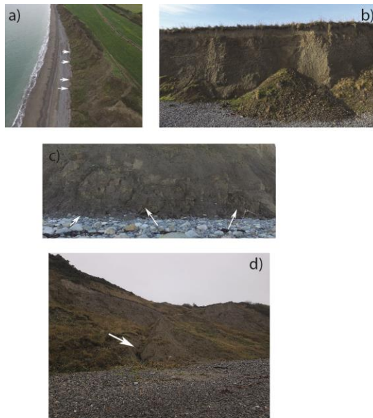
Figure 4: Examples of typical landslides found at site B. a) debris flows; b) Debris falls; c) slumps (small) arrow to left is location of mud flows; d) slump (large)
