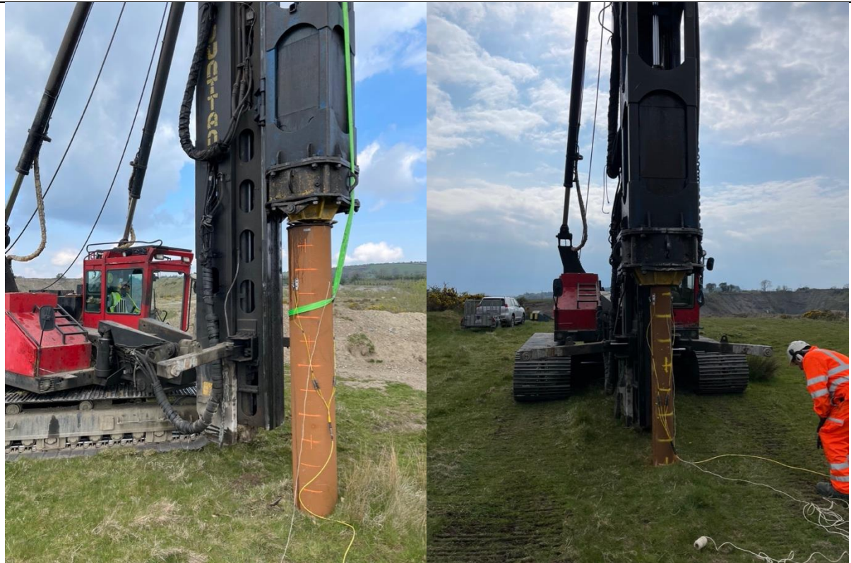
Figure 9: Installation of (a) 457mm diameter and (b) 212mm diameter steel piles in Blessington including pile driving monitoring instrumentation
