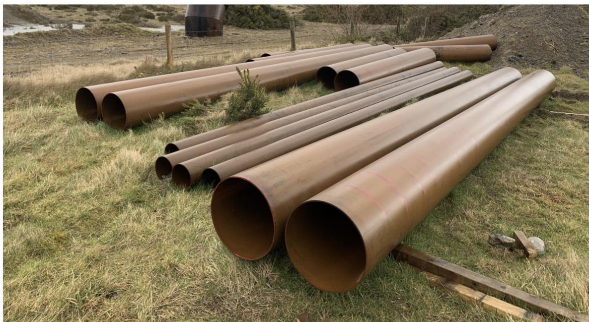
Figure 8: Open-ended steel piles used in testing
