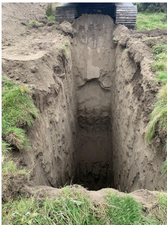
Figure 3: Trial pit at Blessington Site 3 (from Gallagher 2022)
