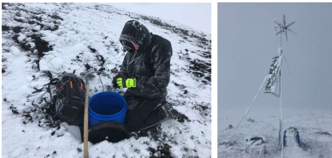
Figure 9 left: installing HS2 at Hekla summit, right: frozen over wind charger at HS1 two days after it had been installed.
