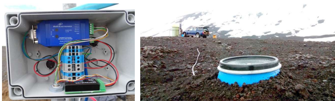
Figure 8 left: field box containing the black DC/DC power and the blue RS232/422 converter, right: installation site of HN1 on top of Litla Hekla at 953m elevation, in the background the green hut used for housing of batteries and electronics.
