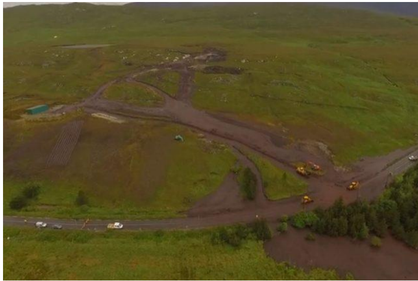
Figure 2 Examples of landslide in Ireland in the last decade: a) the remains of Leenaun bridge after it was destroyed by a debris flow in 2007 (source: rte.ie), b) one of many landslides damaging local road infrastructure during heavy storms in December 2013 (author's photo of Dog's Bay, Co. Galway), c) landslide and coastal erosion of a coastal cliff supporting rail infrastructure in Co. Wicklow in 2016 (source: Skycam Ireland), d) peat slide blocking a national road N59 in Co. Galway in 2016 (source: blogs.agu.org/landslideblog )
