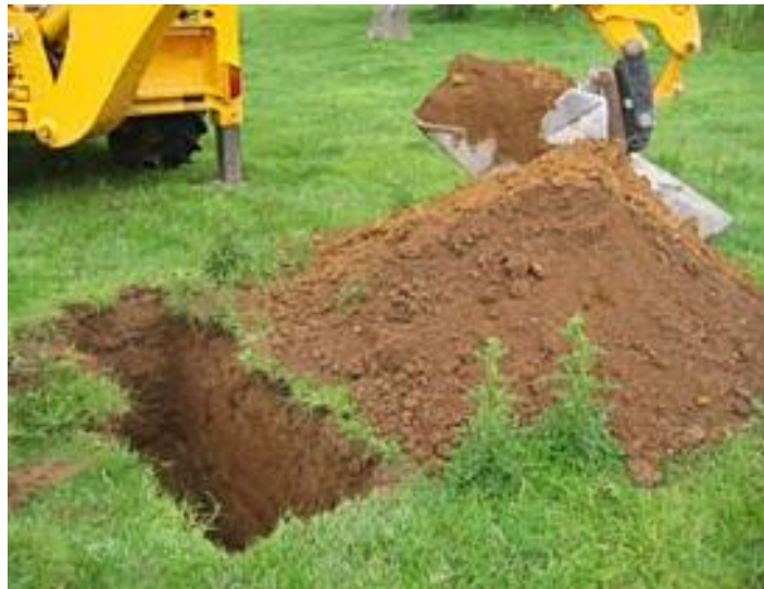
Figure 29 Trial Pit ( http://www.wilson-bailey.co.uk/ ).
