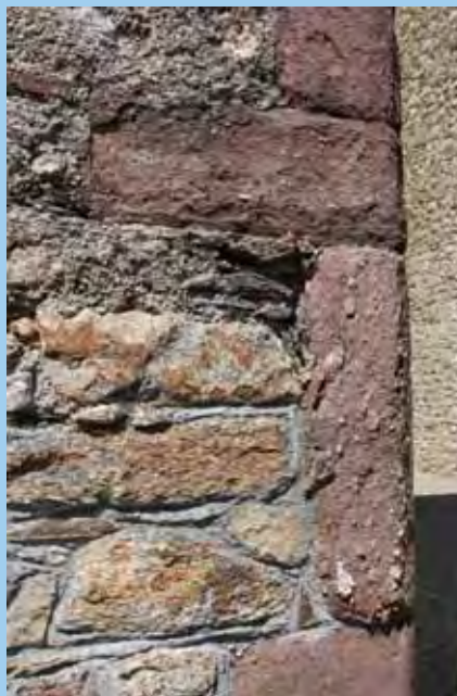
Detail of the cornerstones where quartz pebbles can be seen
